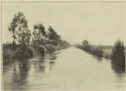
MAIN IRRIGATION CANAL
